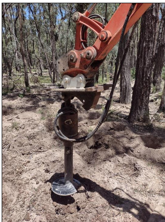
Plate 2.5 Excavator with auger attachment drilling holes for plants.
