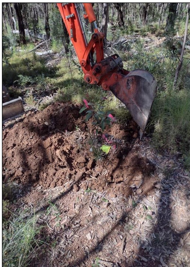
Plate 2.3 Mechanical extraction using small excavator.
