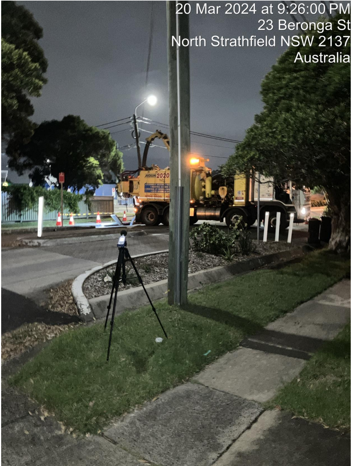
Attended Noise Monitoring Rion-42- 23 Beronga St, North Strathfield.
